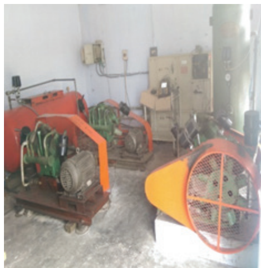
Figure 40: Reciprocating Compressor
