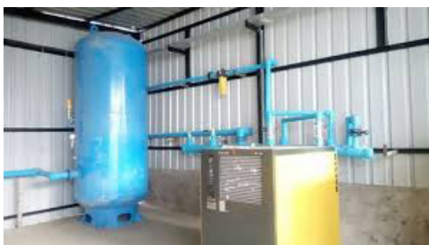
Figure 42: HDPE Aluminum Pipeline
