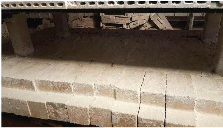
Figure 68: Existing high thermal mass refractory in kiln car
