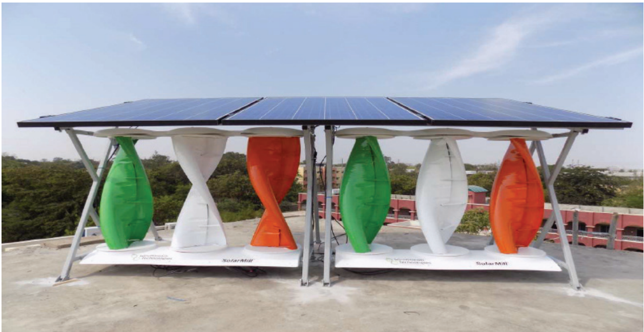
Figure 83: Solar-wind hybrid system
