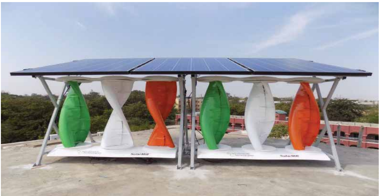
Figure 43: Solar wind hybrid system
