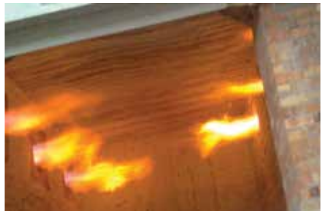
Figure 50: Improper air to fuel ratio
