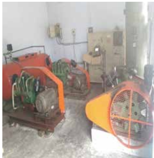
Figure 30: Reciprocating Compressor
