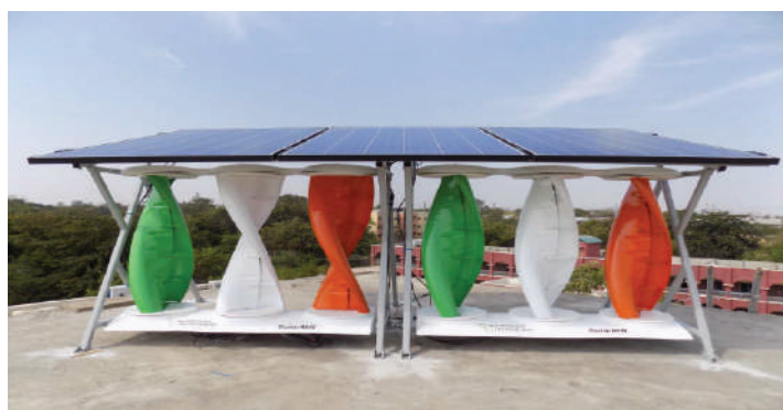
Figure 22: Solar Wind Hybrid System
