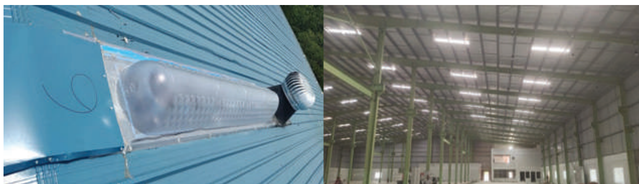
Figure 30: Light Pipe Installation
